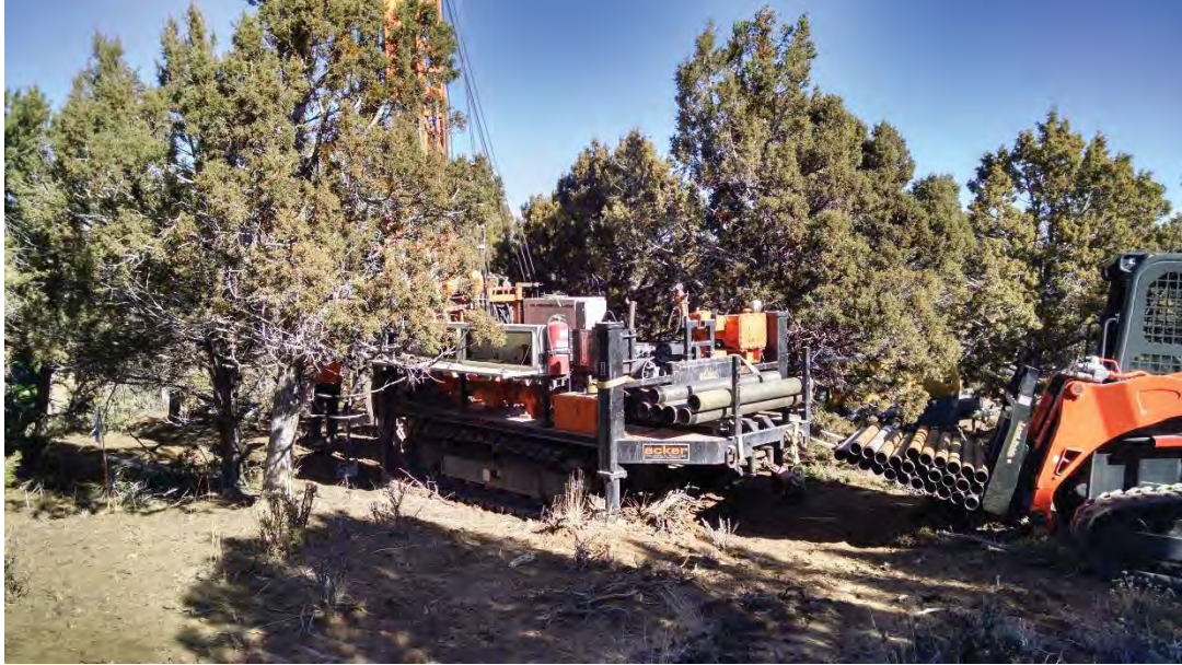
Acker Track Rig at Boring A-1
