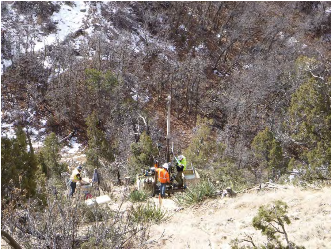
Portable Viper Rig at Boring B1-10
