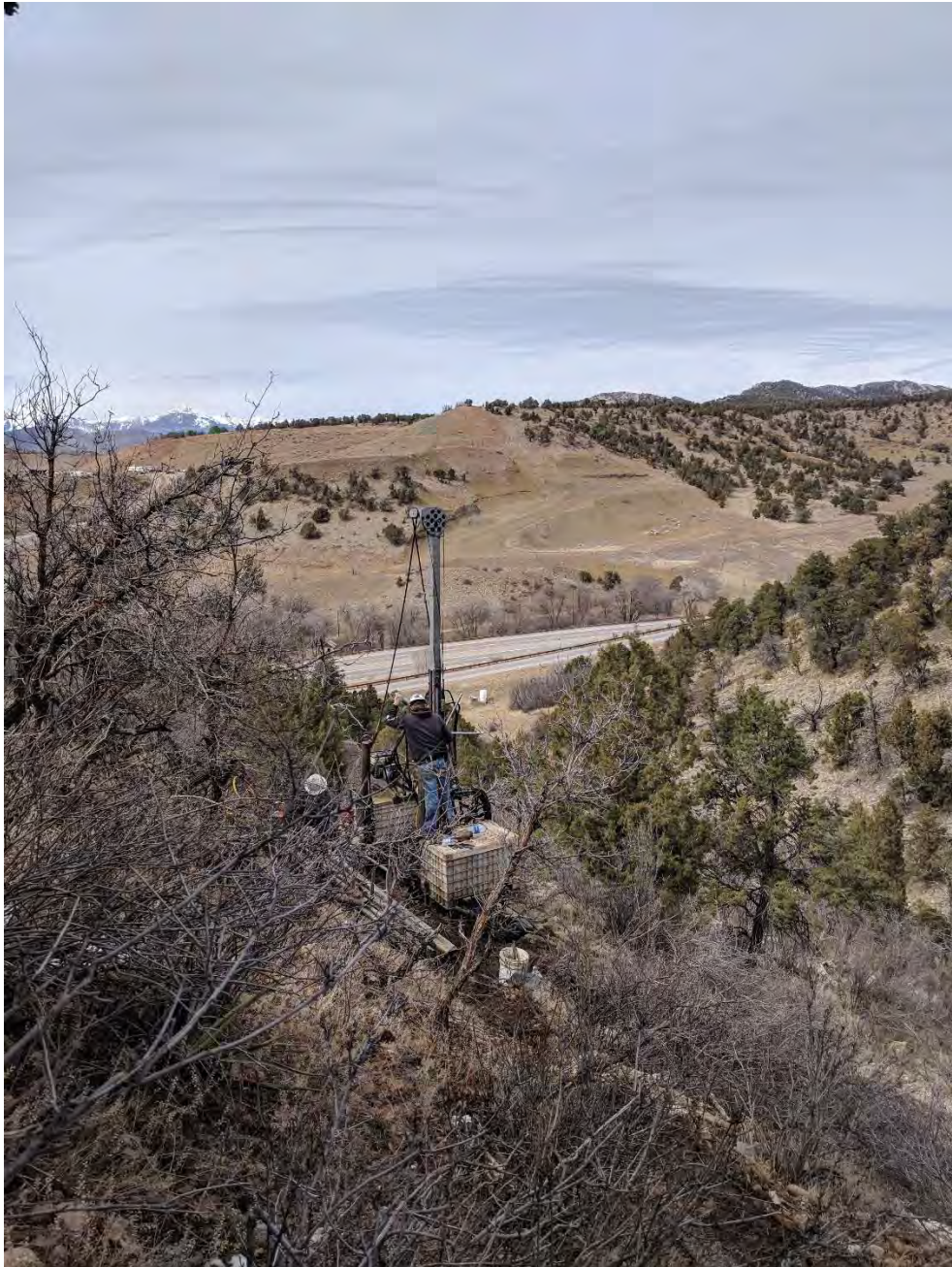
Portable Viper Rig at Boring B1-04
