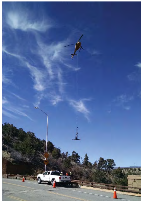
Helicopter Placing Portable Rig at Boring D-01
